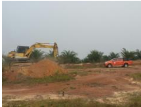
Figure 4. On Progress Activity
