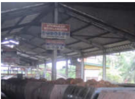
Plate 1: Hazard and PPE signage at the Kerteh POM sterilizer area that included PPE for noise.
