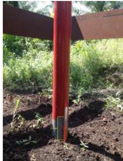
Picture 2. Subsidence pole No. 6 in Block 16A Phase 2, PHP-1 Estate
