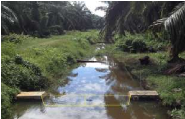
Picture 1. Bund Off No. 19 in Block 15C Phase 2, PHP-1 Estate
