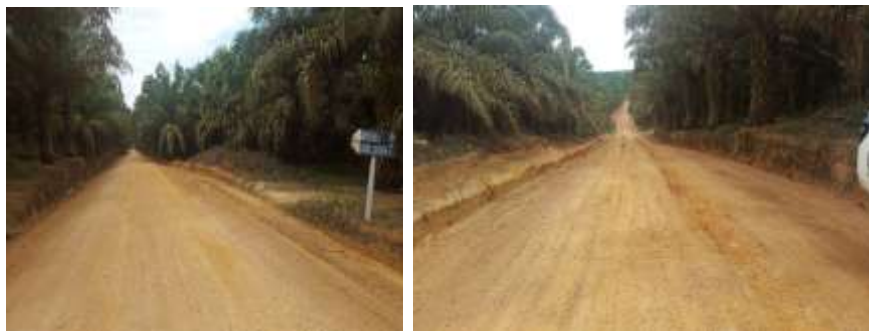
Road condition in LJ1 and LJ2 estate
